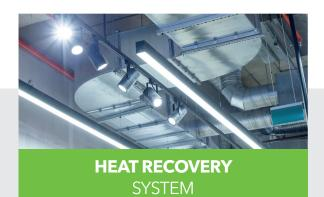
A heat recovery system is installed at the facilities. The heat so recovered is used for space heating. Heat is recovered from two sources: the ventilation system and exhaust air from presses.
