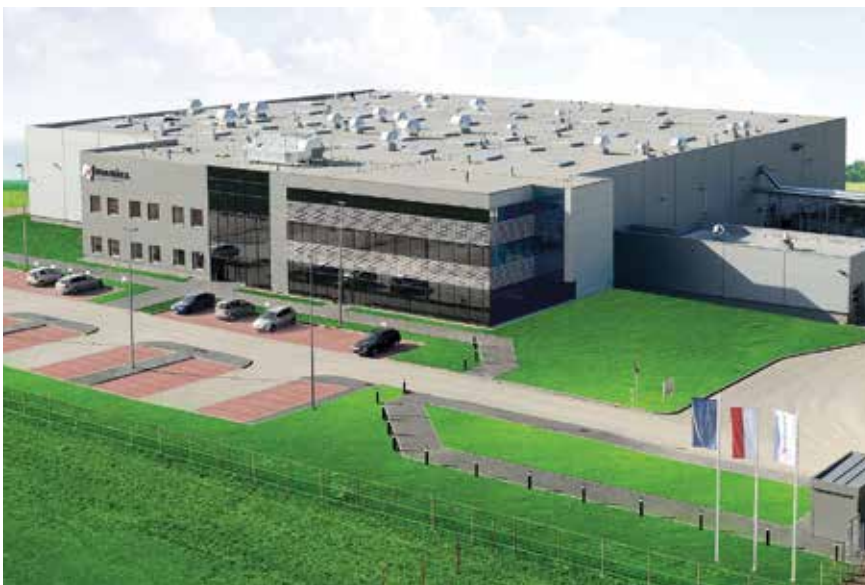
The new headquarters is a typical Greenfield project, located just over a kilometre from built-up areas, but only 3km from access to the A2 motorway. It is one of the most modern plants in Europe dedicated to producing packaging for the food, pharmaceutical and cosmetics industries.
